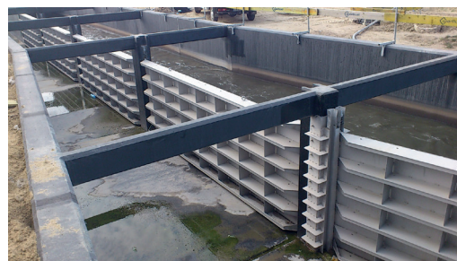
4x stop gates 5000 mm x 2000 mm wastewater treatment plant Warsaw, Poland
