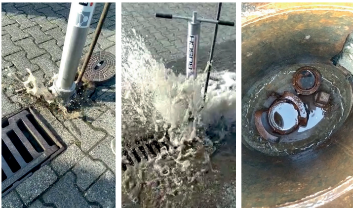
Surface box cleaning with BÜSCH Surface box cleaner made of stainless steel
