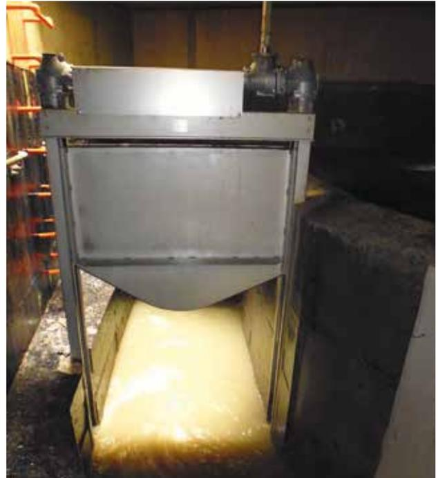
CP3-RS channel penstock 3-side sealing 1800 x 1200 mm as two-spindle version, both spindles located outside in the frame, not in the direct media flow
