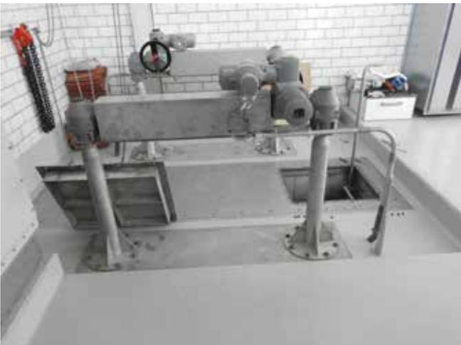
Two XL4 penstocks 2000 x 1300 mm as two-spindle version, penstock bridges with mounted gear boxes and actuator, located over floor
