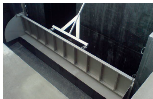
Overfall weir 5000 x 800 mm wastewater treatment plant Czajka, Warsaw
