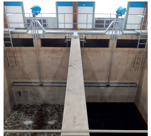
Double rotary weir with front control with electric drive. Wastewater treatment plant, Germany
