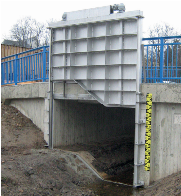
Penstock with adapted flume at the bottom
