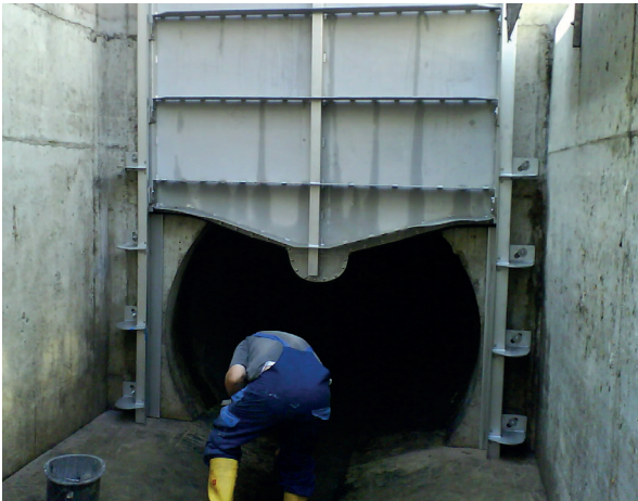
Penstocks with adapted channel bottom
