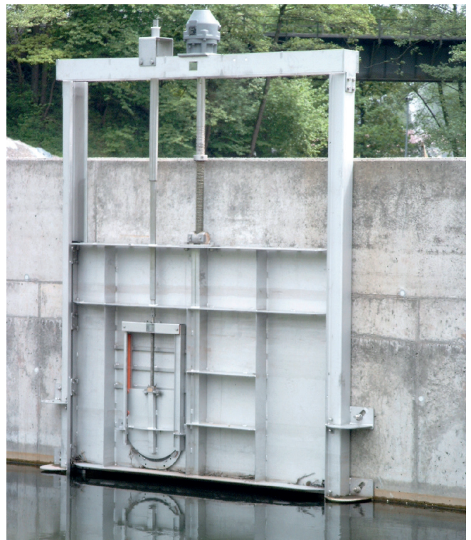
High water penstock allows taking cooling water
