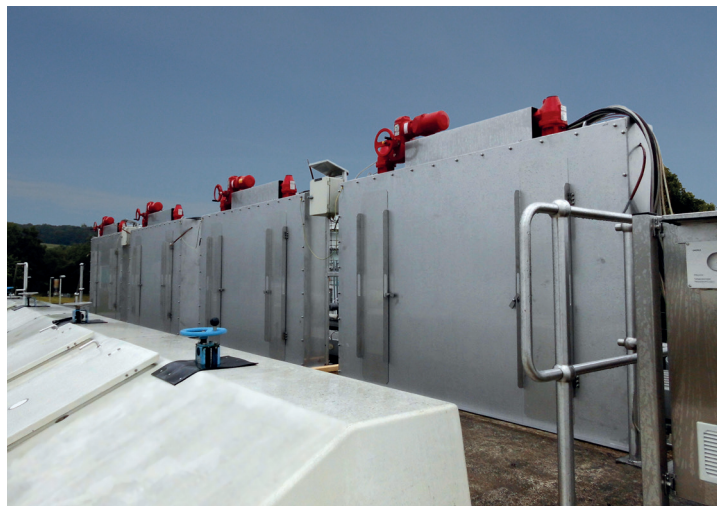
Housing for penstocks to protect penstocks protruding out of the building
