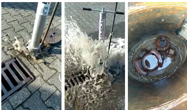
Street cap cleaning with BÜSCH Street cap cleaner made of stainless steel
