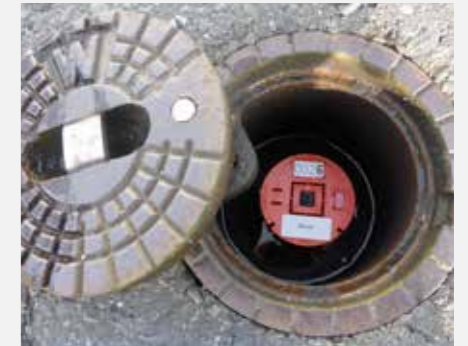
ID-Fix installed on house connection
